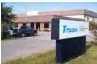
US Tsubaki Portland Plant
