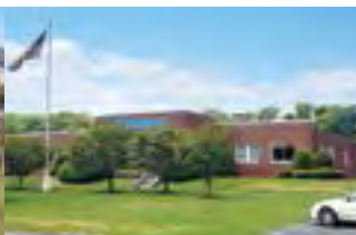
US Tsubaki Holyoke Plant
