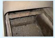
Fly Ash Conveyor: Dust Conveyor Under Boiler
